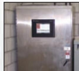
Optional programmable logic controller continuously monitors and controls UV system functions. Interfaces with power distribution center(s), UV reactor(s), influent water temperature sensor, flow meter, hydrogen peroxide delivery system, and any valves (optional).
